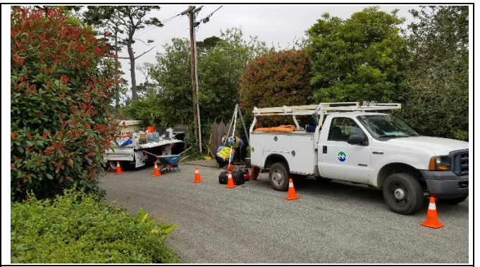
Photo: Pipe Repairs
