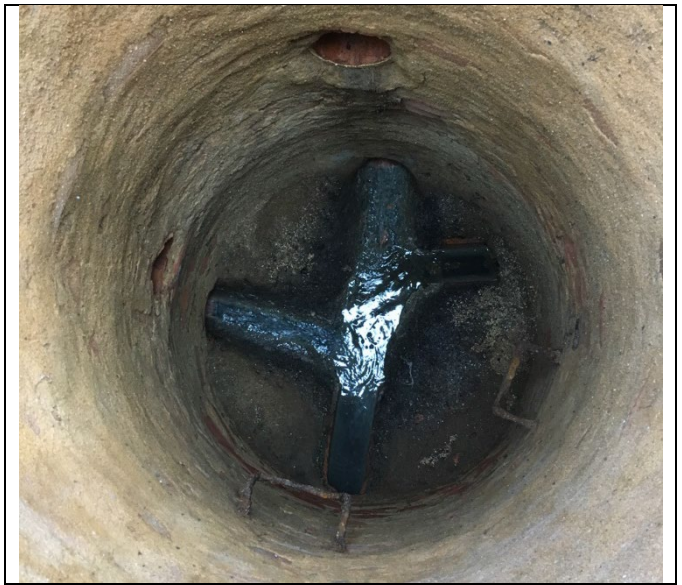
Photo: Inside of Sewer Manhole
