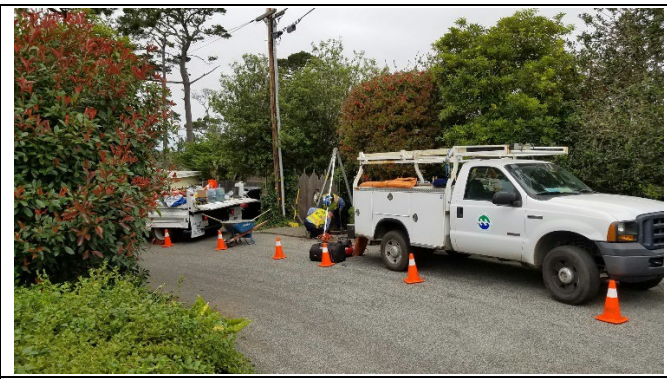
Photo: Pipe Repairs
