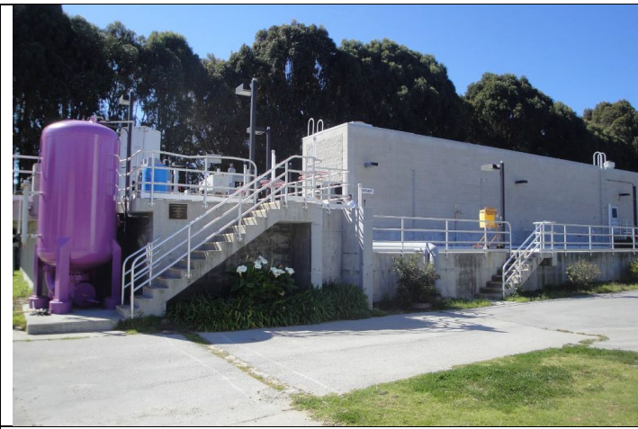
Photo: Exterior of Tertiary Building
