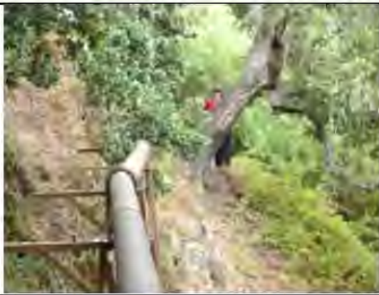
Photo: View gravity pipe in Carmel easement
