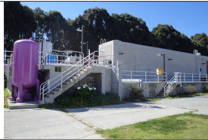
Photo: Exterior of Tertiary Building
