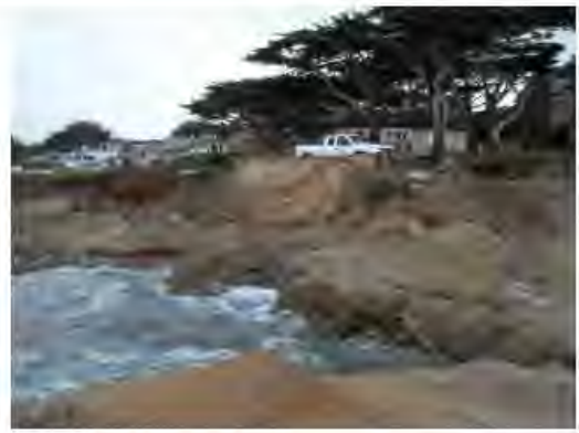
Photo: Looking at Pump Station Exterior
