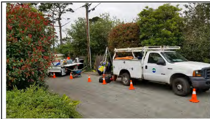
Photo: Pipe Repairs
