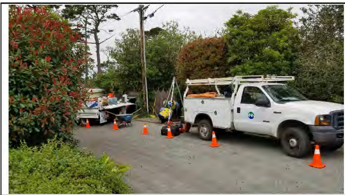
Photo: Pipe Repairs
