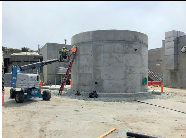
Photo: New Sludge Tank Under Construction
