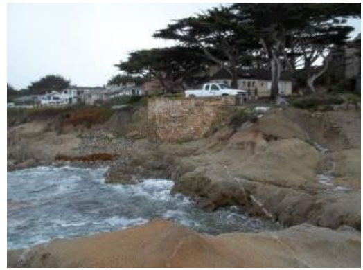
Photo: Looking at Pump Station Exterior
