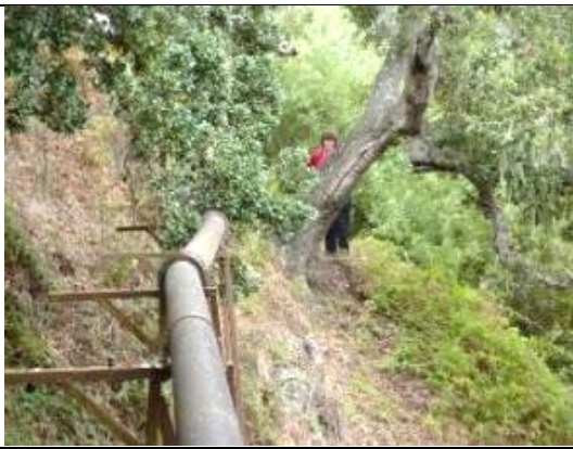
Photo: View gravity pipe in Carmel easement
